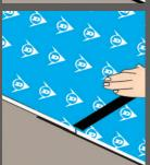
All seams must be sealed with a waterproof tape\* to ensure no moisture can pass through.
