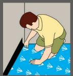
Roll out the selected Dunlop hard flooring underlay and trim any excess so that the ends and sides fit neatly against all walls.
